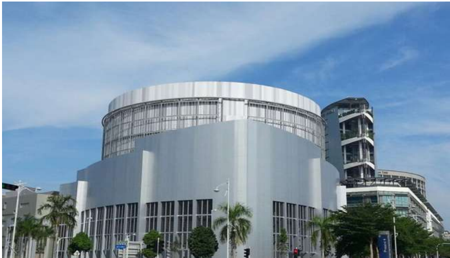
Gas District Cooling Plant - Putrajaya
