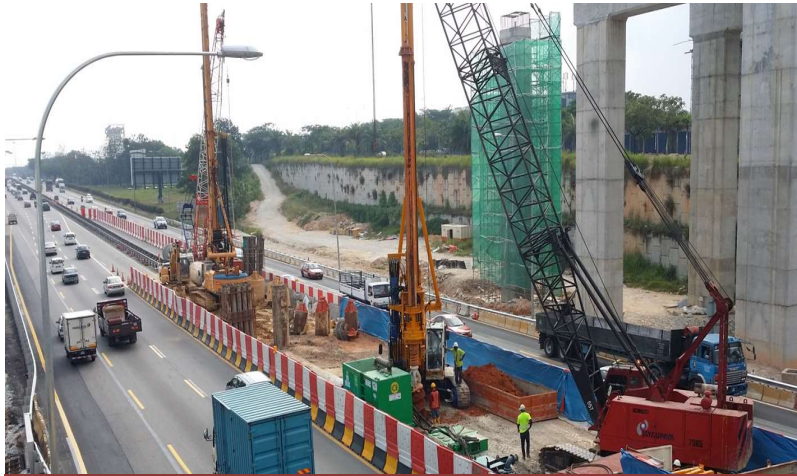
Pile Foundation Works
