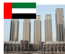
Phase 1, Plot 1 Al-Reem Island Completed: 2009 Value: US$362 mil
